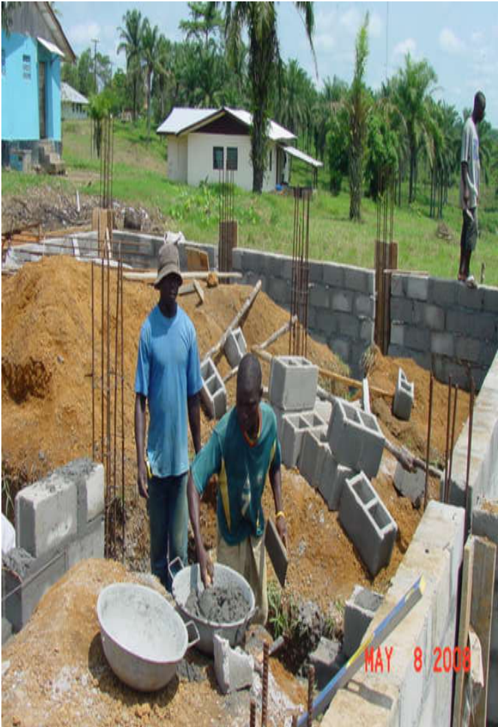
COLLEGE OF BWI UNDER CONSTRUCTION
