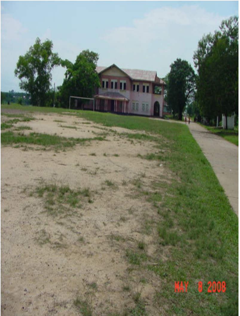
DINNING HALL AND AUDITORIUM ON BWI CAMPUS
